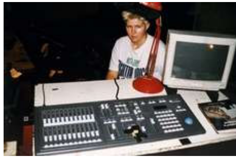
A lighting control desk
